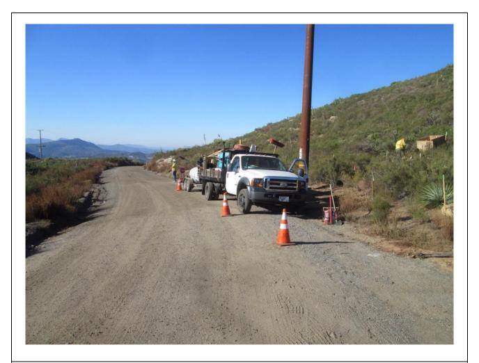
**Photo 6:** During anchor hole drilling at P172692, a traffic control flagperson and cones were stationed to direct traffic around equipment staged on Viejas Grande Road in accordance with APM-TRANS-02 (C 78).
