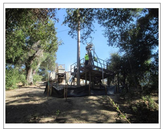
**Photo 3:** A silt fence was observed around the downslope side of the micropile drilling workspace at Z118123 in accordance with the SWPPP (TL 682).
