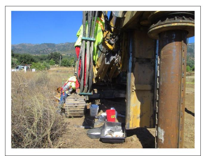
**Photo 5:** During direct bury pole hole drilling at Z118049, the crew stopped drilling to respond to an equipment leak in accordance with the Spill Response and Notification Plan (MM-PHS-2) (TL 682).
